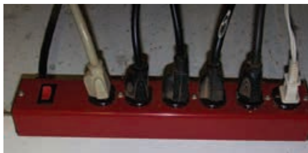
Figure 2-19. When too many tools or machines are drawing current from the same circuit, the circuit can become overloaded. The result can be a tripped circuit breaker or even a fire.
