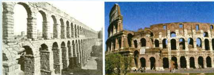
Reminders of the Roman Empire. Left: Built in the first century A.D., this Roman aqueduct still brings water to the city of Segovia, Spain, from a river 10 miles (16 km) away. Only about 900 feet (274 m) of the aqueduct is above the ground; the rest consists of underground water conduits. This photograph shows some of the 148 arches needed to span uneven terrain so that water can flow by gravity. Right: The Colosseum at Rome. This huge amphitheater was built around A.D. 80, and its outer shell still stands today. During the Roman persecutions, thousands of Christians were killed here for public entertainment.
